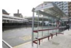
Bus shelters at Leeds Station interchange
